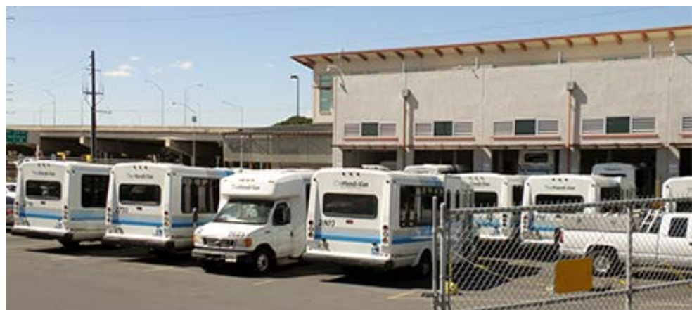
The Handi-Van base and maintenance yard on Middle Street has an estimated capacity to handle between 185-195 paratransit vehicles. The facility is nearing capacity with the current fleet of 181 Handi-Vans, with no room to expand.
