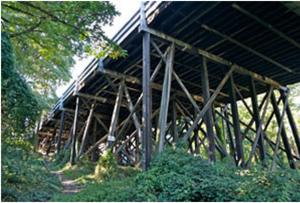
NE 45 th St Viaduct
